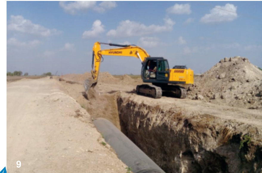
Trench Backfilling Work
