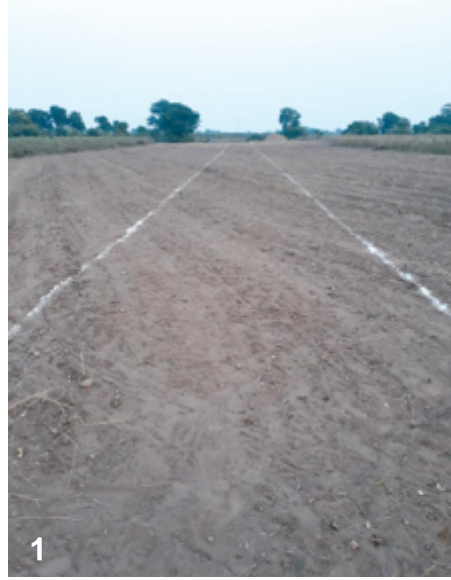
Line Marking and Excavation Work
