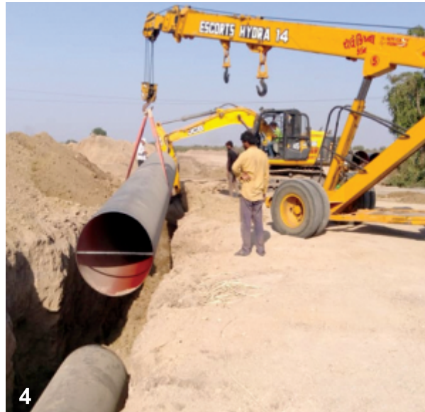
Pipe Laying Work
