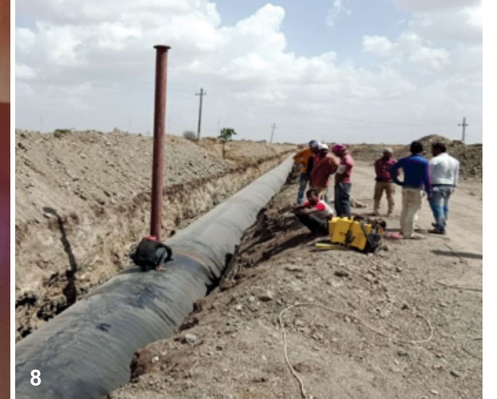
Air vent pipe erection work is in progress
