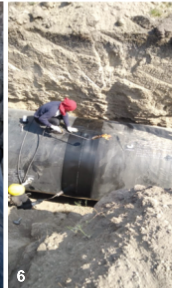
Outer Joint Coating
