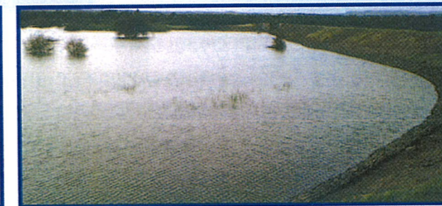
Water filled up due to rains
