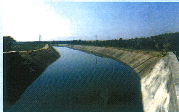
Canal Rehabilitation Work
