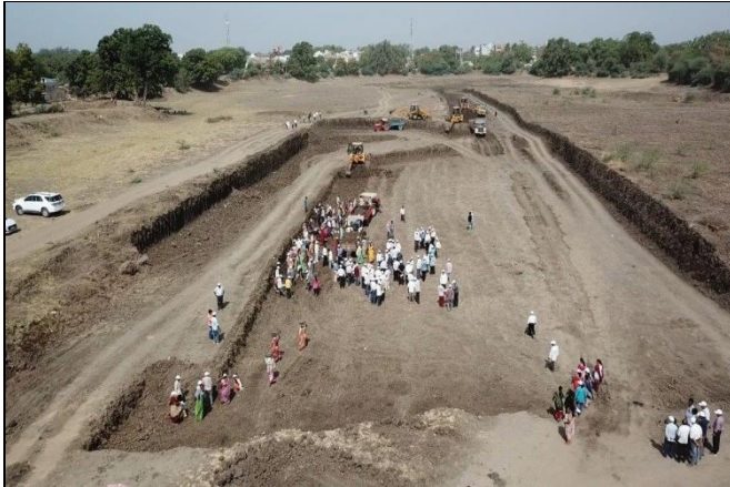
Work in Progress Deepening of Pond
