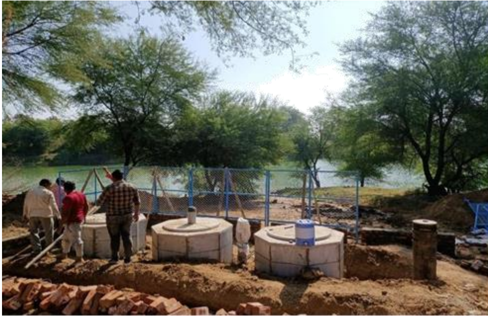
Figure 18-Artificial Recharge System under construction - Atal Bhujal Yojana
