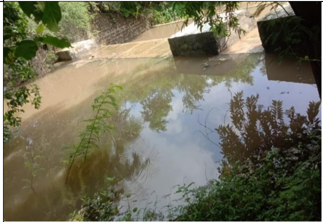
Check dam Construction
