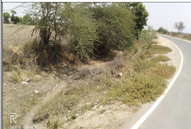
Cleaning of Drain - Before
