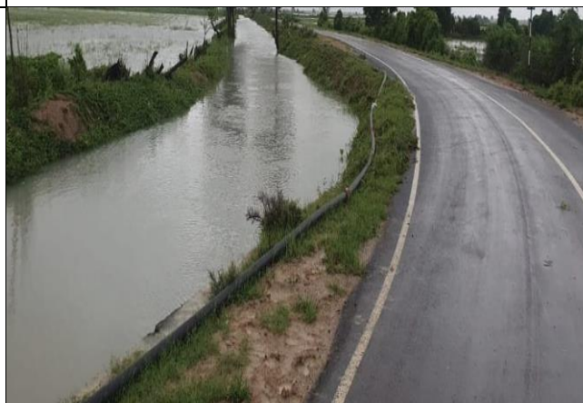
Cleaning of Drain - After
