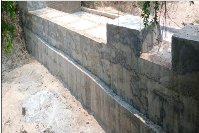
Built up check dam Water storage in Check dam
